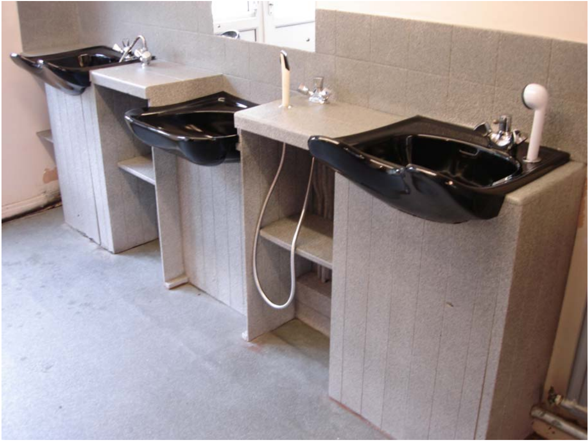
Fig1: Basins re-enamelled in high-gloss black and panels resurfaced in stone fleck granite effect
