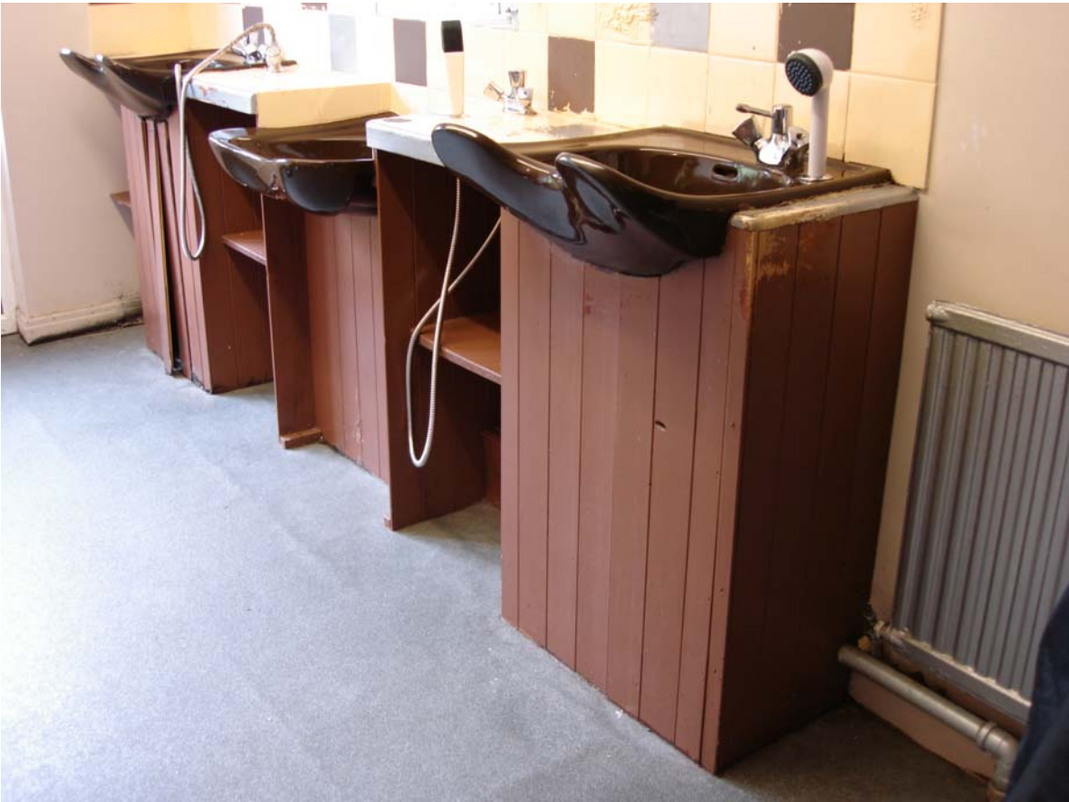
Fig1: Basins re-enamelled in high-gloss black and panels resurfaced in stone fleck granite effect
